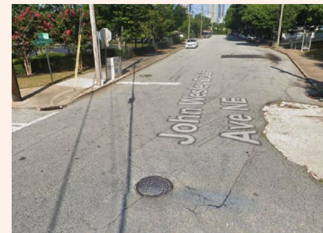
5 Key trail crossing is not prominently marked.
