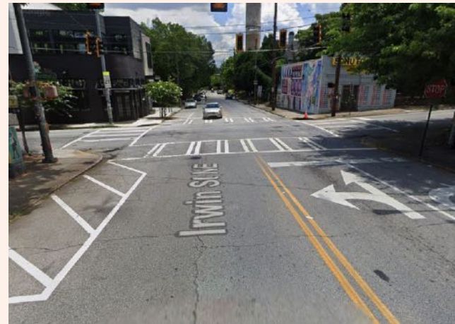
10 Excess pavement at intersection due to on-street parking lanes.
