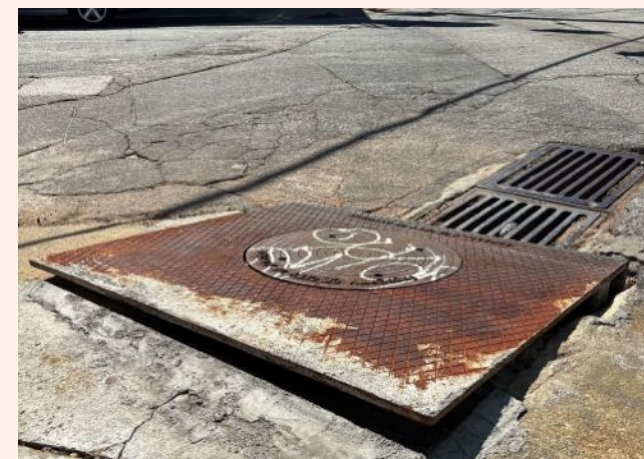
20 Obstacles related to utility infrastructure; stones in tree wells and abandoned bioswale wash downstream into Irwin intersection and create crosswalk obstacles.
