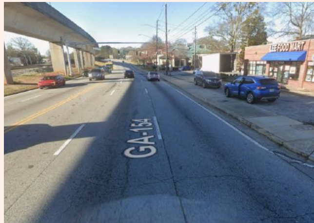
7 Uncomfortable walking and biking environment along Lee St, a five-lane roadway.
