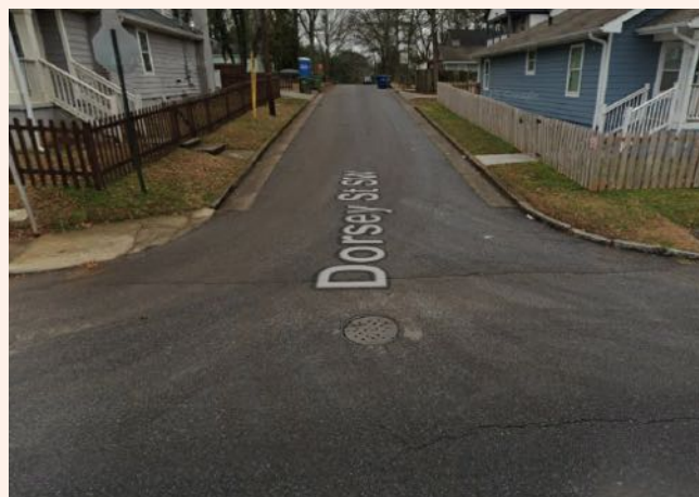
21 Missing sidewalk ramps at Oakland Ln SW/ Dorsey St SW.
