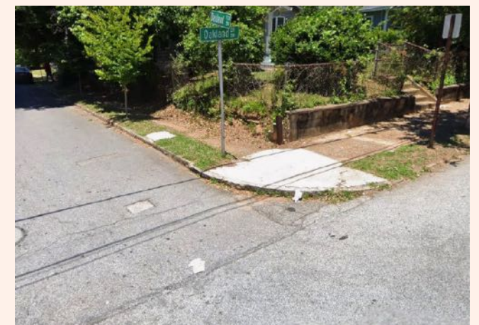
17 Missing sidewalk ramps on Oakland Dr SW/Oakland Terrace SW.
