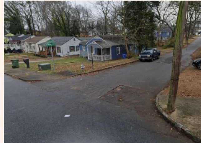
6 Missing sidewalks and ramps on Wilmington Ave SW.
