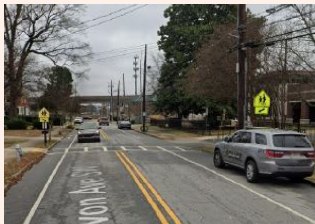
9 Existing crossing near school on Avon Ave SW needs safety improvements.
