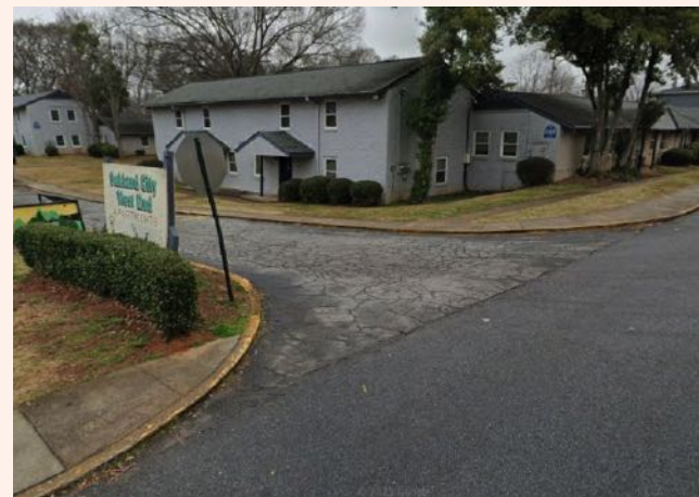
20 Missing sidewalk ramps at Oakland Ln SW/ Driveway to Oakland City West End Apartments.
