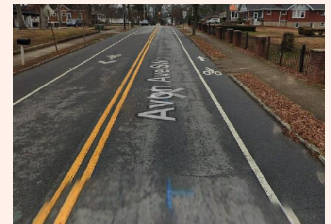
4 Bike lane on Avon Ave SW is too narrow and substandard.
