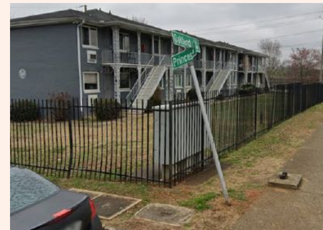
26 Damaged street sign post Princess Ave SW/ Oakland Ln SW.
