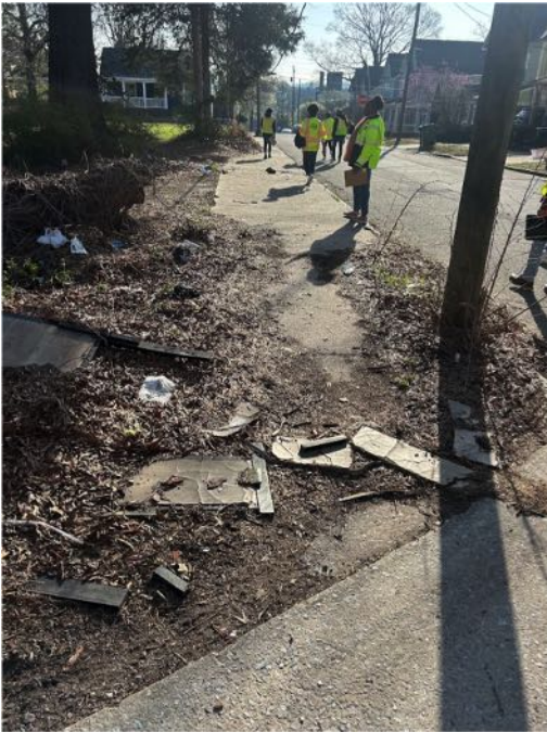
PHOTO 11: TRASH AND DEBRIS ON THE SIDEWALK ALONG GLENN STREET
