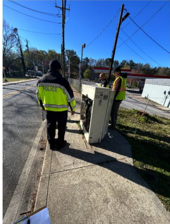
PHOTO 4: EXPOSED AT&T BOX IN THE SIDEWALK ALONG OLD HAPEVILLE ROAD
