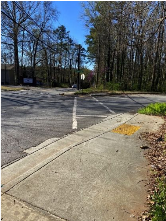
PHOTO 7: OLD HAPEVILLE ROAD AT HAPEVILLE ROAD
