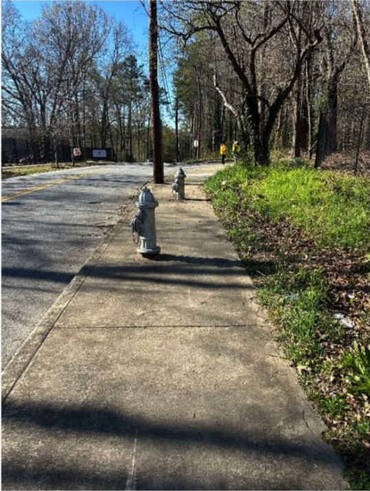
PHOTO 5: FIRE HYDRANTS AND UTILITY POLES IN SIDEWALK ALONG OLD HAPEVILLE ROAD
