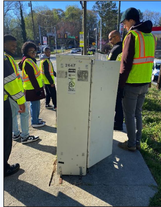
Utility obstruction located in the sidewalk south of Old Hapeville Road with exposed wiring.
