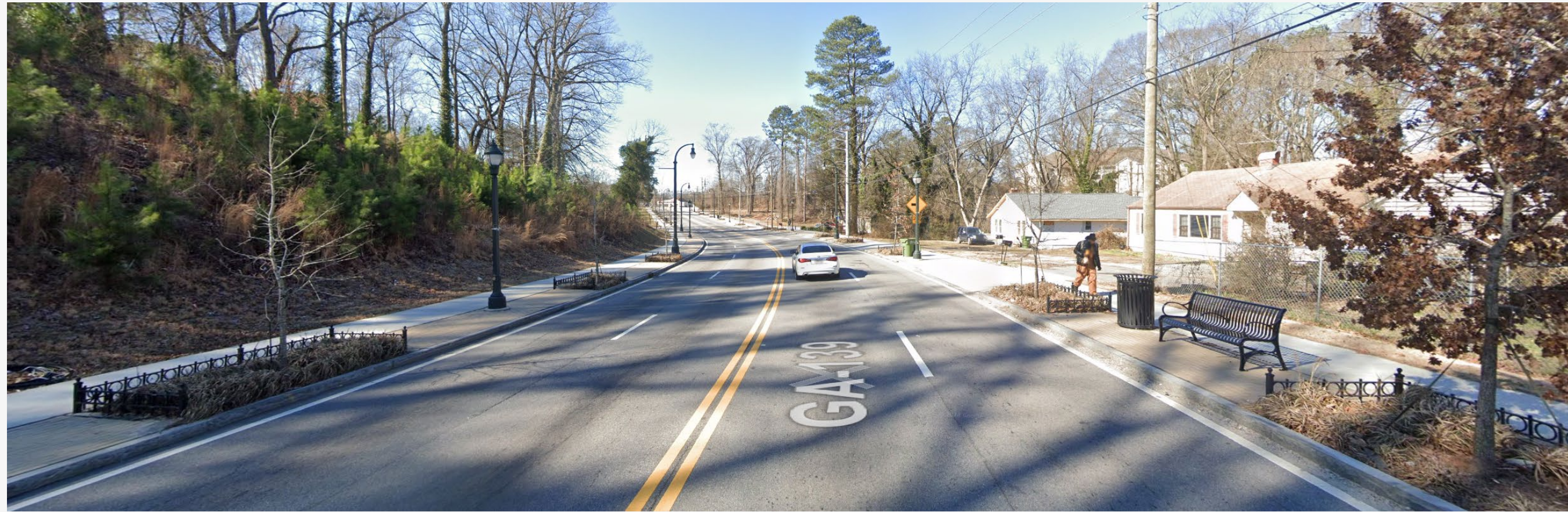
Figure 1: MLK Jr. Dr SW (SR 139) looking west
