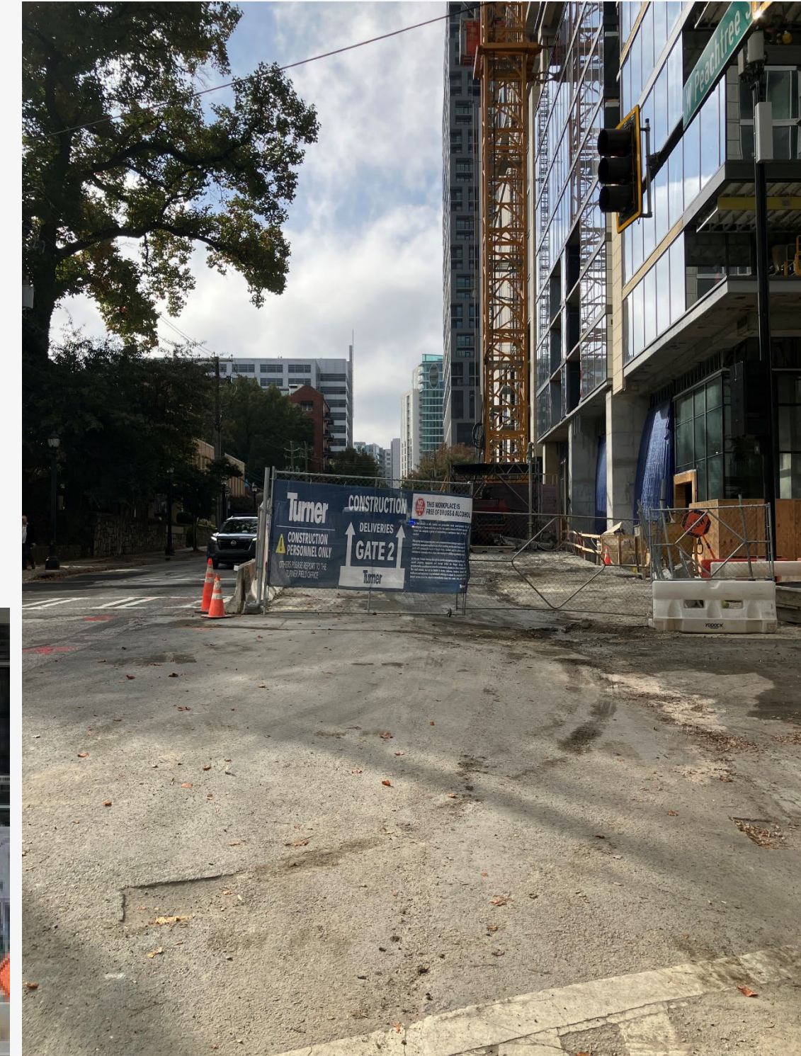
Figure 3: West Peachtree NW looking north construction gate
