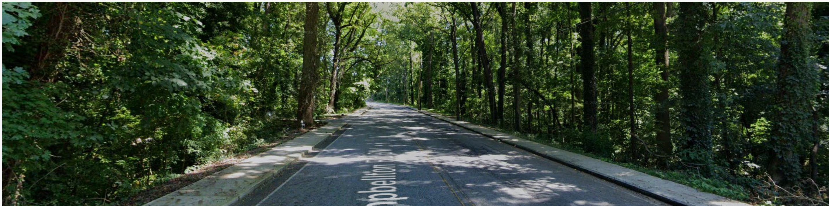
Figure 2: Campbellton Rd SW at Wells Dr SW looking east
