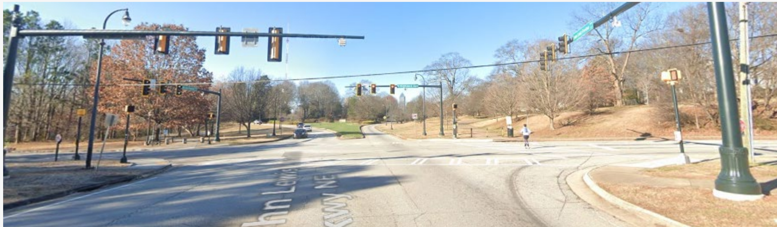
Figure 2: Freedom Parkway (SR 10) looking west
