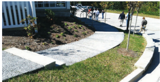
Pervious concrete sidewalk in Chattanooga, TN
