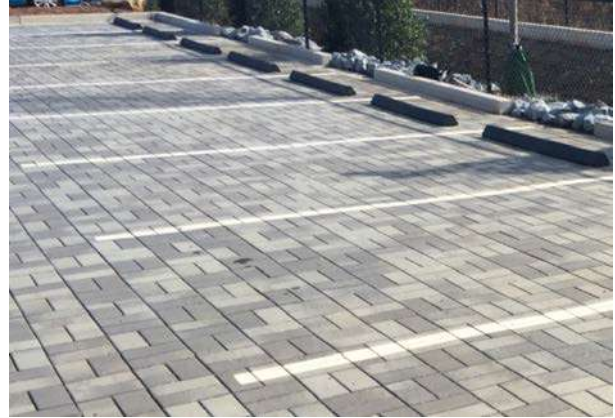
Permeable pavers used for parking lot
