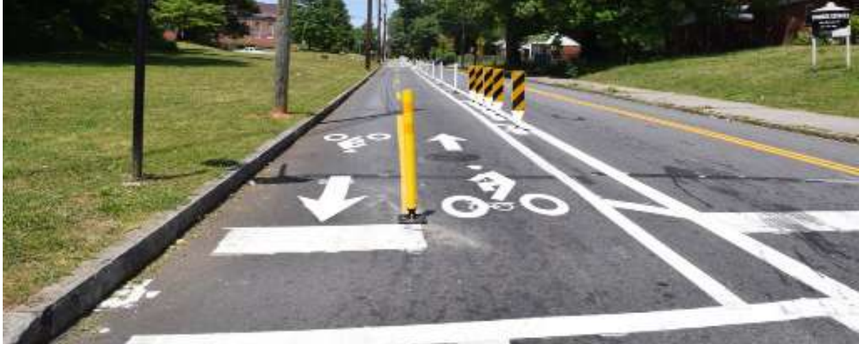
The Westview Drive two way protected bicycle facility was installed during a typical resurfacing project.
