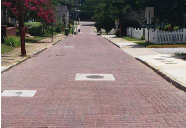
Permeable pavers used for low-speed roadway
