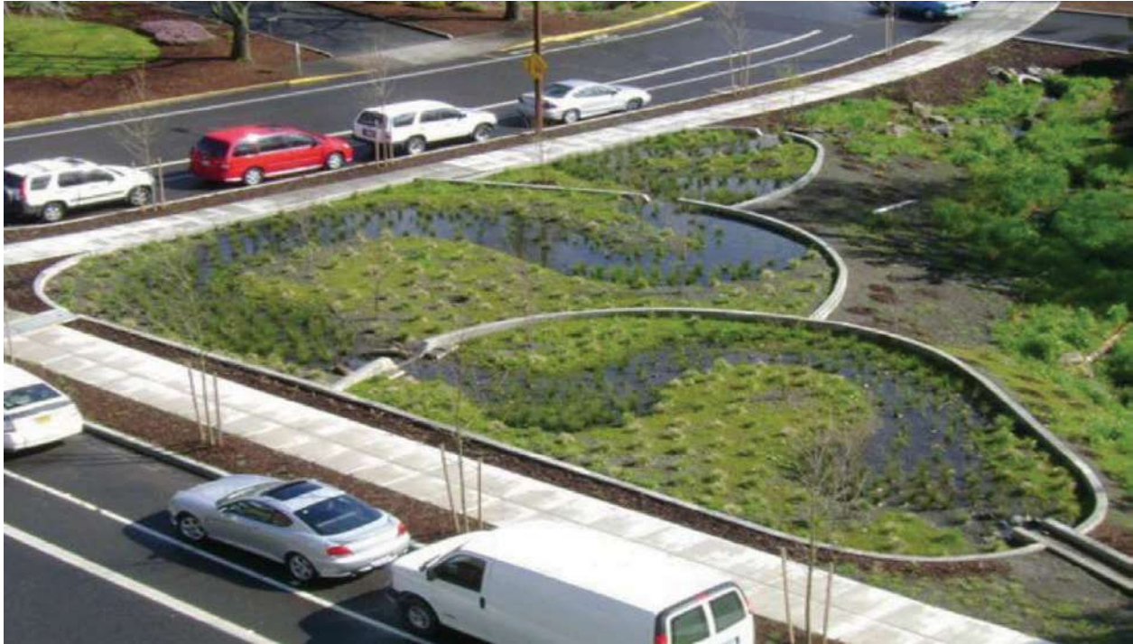
Larger roadside bioretention (Credit: City of Portland, OR)
