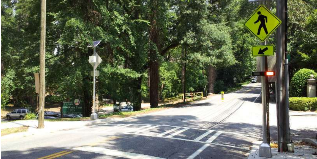
Rectangular rapid-flash beacon, Peachtree Dunwoody Road
