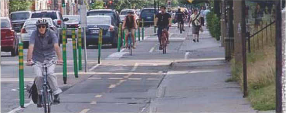
The two-way cycle track along 10th Street will provide a direct, on-street bikeway connection from the Eastside Trail to Piedmont Park and Midtown. When completed, it will function similarly to the two-way cycle track above with a buffer and bollards separating cyclists from motor vehicles.
